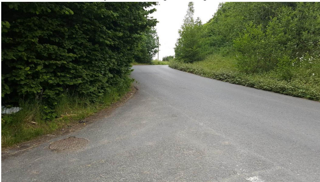
Plate 12.4 L6026 / local road junction – looking west along L6026
