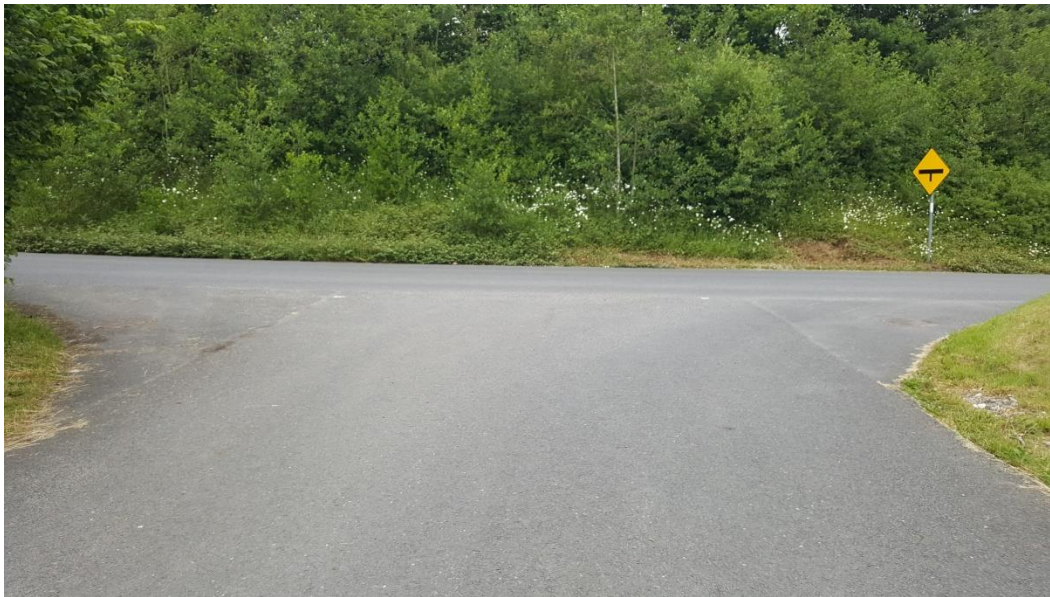
Plate 12.6 L6026 / local road junction – looking north towards L6026
